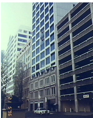
Figure 6 View of along Sussex Street (1996)
