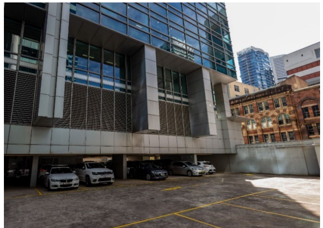
Figure 14 View from the Level 6 (existing car park) looking north-east
