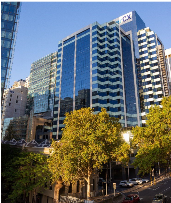
Figure 20 View of 2 Market Street looking north-east
