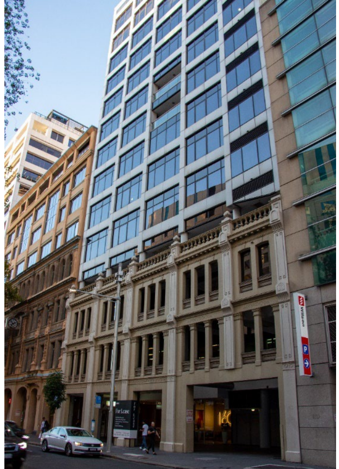
Figure 18 View along Sussex Street to the north
