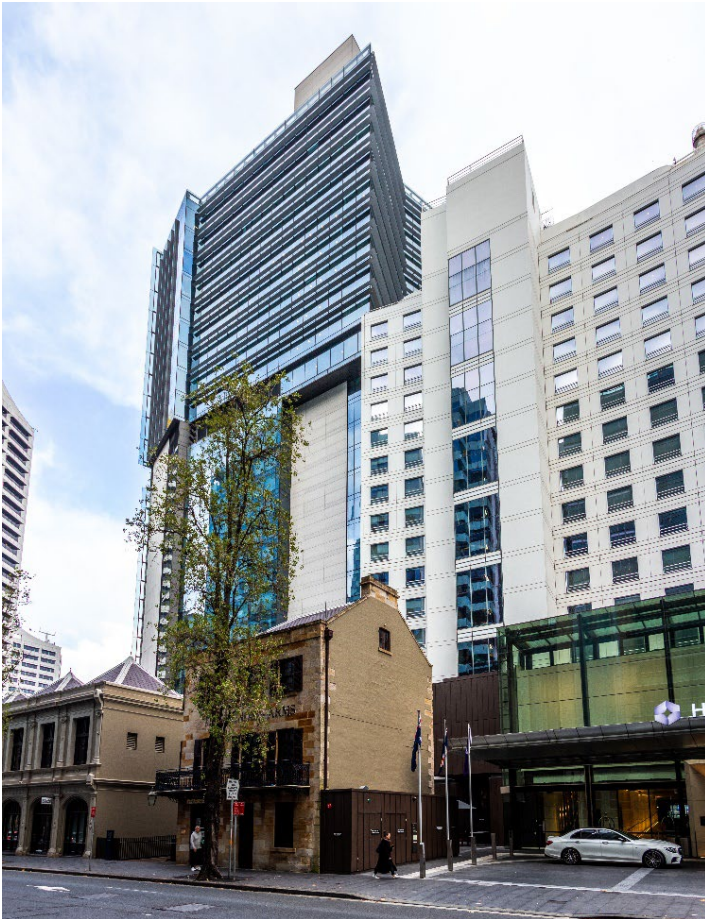
Figure 24 View of The Dundee Arms and Hyatt Regency looking south-west
