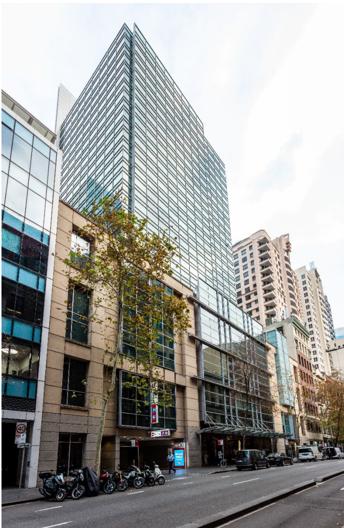
Figure 8 View from Kent Street looking north-west
