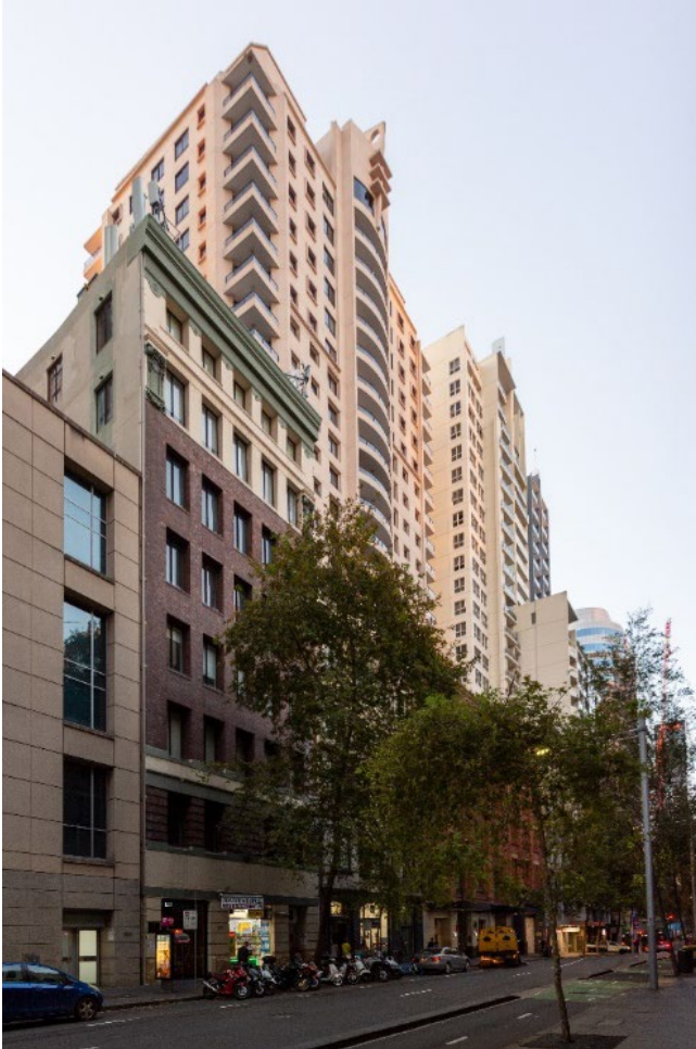
Figure 17 View along Kent Street to the north
